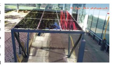
frameless solar modules. One of the two solar micro systems is installed on the roof of the building, to supply the building with electricity and provides partial shading from the direct sunlight coming through glass. The second solar power plant which provides electricity to the charging terminal of electric vehicles is installed next to the building, on the roof of a small parking type construction.
